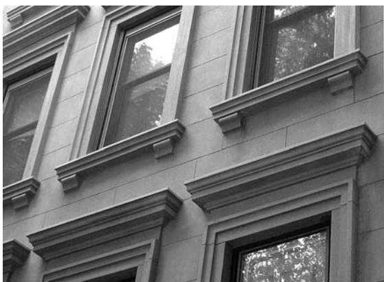
Detail of 158 East 74th Street showing footed sills
